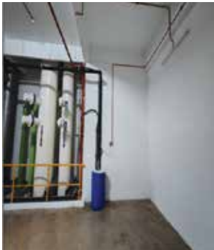
Recycle of cooling water from air-conditioning systems for use in cooling towers
