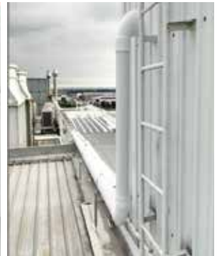
Recycle of rainwater harvesting for use in cooling towers
