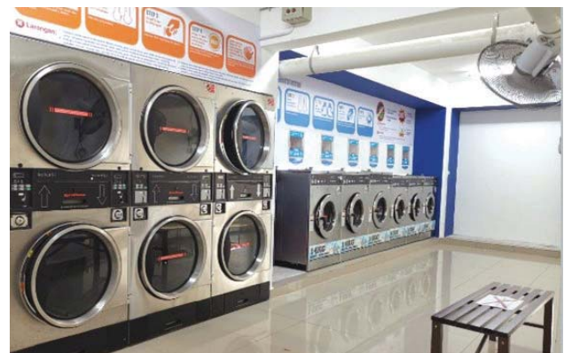
Laundry facilities within the dormitory
